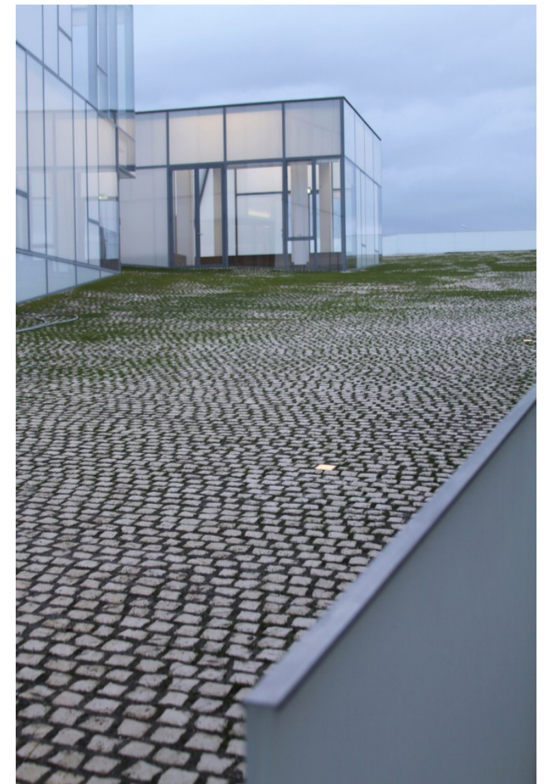
Graded paving treatment to transition between the external platform height and the internal ground level
