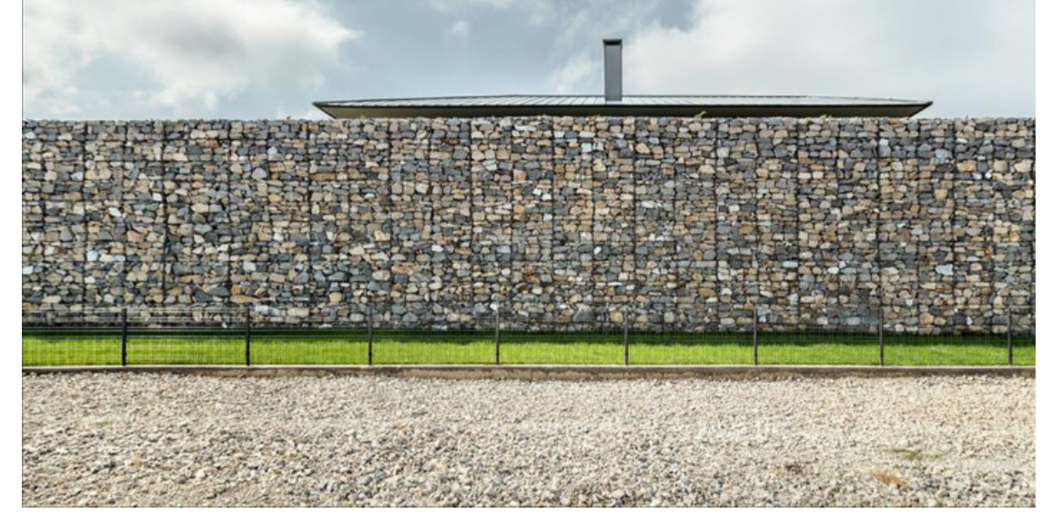
Blue metal filled gabion walls are proposed for areas where soil retention is required. Gabions provide a textural quality and material familiarity that will blend with the railway setting
